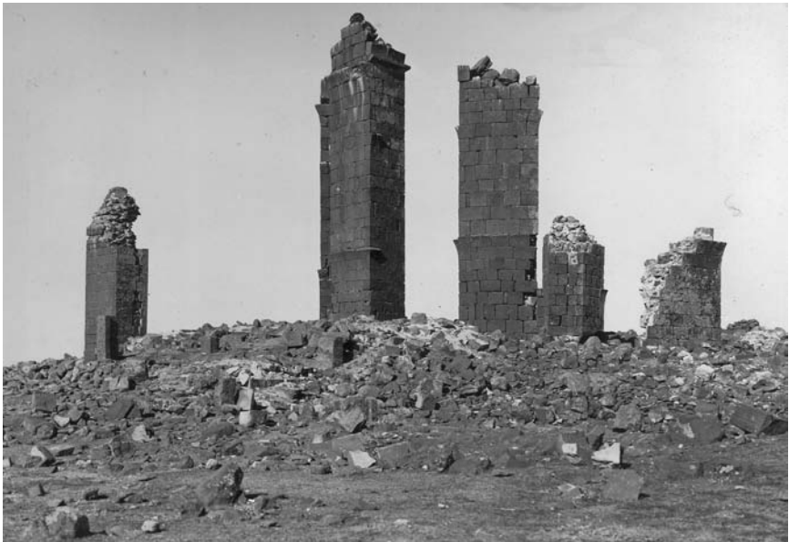
Fig. 2.7.3 Five piers of the Octagon
